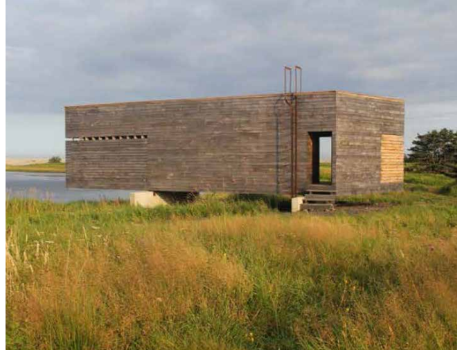
The Village Architect. Shobac Campus, Upper Kingsburg, Nova Scotia, Canada. Photo: © Brian MacKay-Lyons
