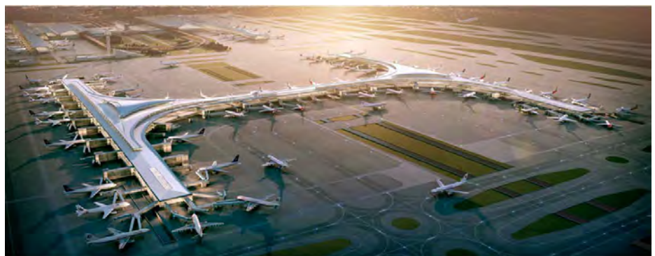
Pudong Airport expansion. Photo courtesy of Otis Elevator.
