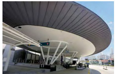
Outram MRT Station
