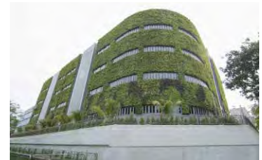
Factory building at Tagore Lane clad with 1500 square metres of Greenology Vertical Greenery panels.
