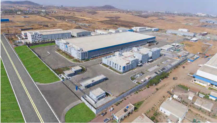
thyssenkrupp's newest Multi-Purpose Facility (MPF) for the elevator industry in Pune.
