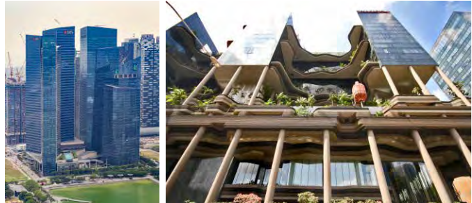
PanU was the sole supplier of Self Compacting Concrete to projects including Marina Bay Financial Centre (left) and PARKROYAL on Pickering hotel (right) in Singapore. Photos: © Pan-United Corporation Ltd
