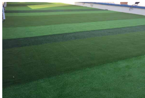
GreenTurf Cool Earth System on the rooftop. Photo: © Advance Sports Technologies Pte Ltd
