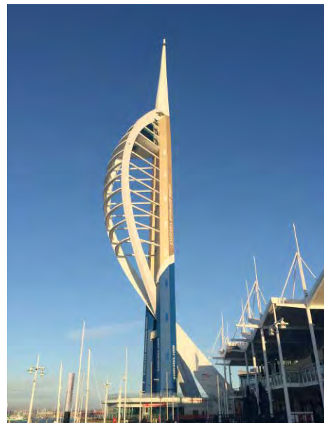
The Emirates Spinnaker Tower in Portsmouth which has been protected with AkzoNobel's steel coatings and Flexcrete's concrete coatings. Photo: © Flexcrete
