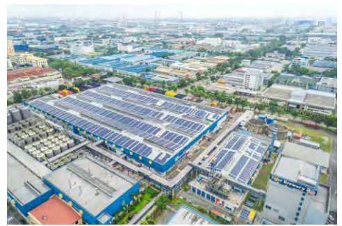
Premises of Asia Pacific Breweries Singapore (APB). Photo: © REC Solar
