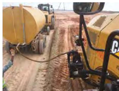
Above and left: A Cat RM500B rotary mixer has also been involved in the construction of a third runway at Singapore Changi Airport.
