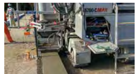
Koyanagawa was tasked to slipform concrete bases for the solar panels to be mounted on. The work had to be completed within 22 days.
