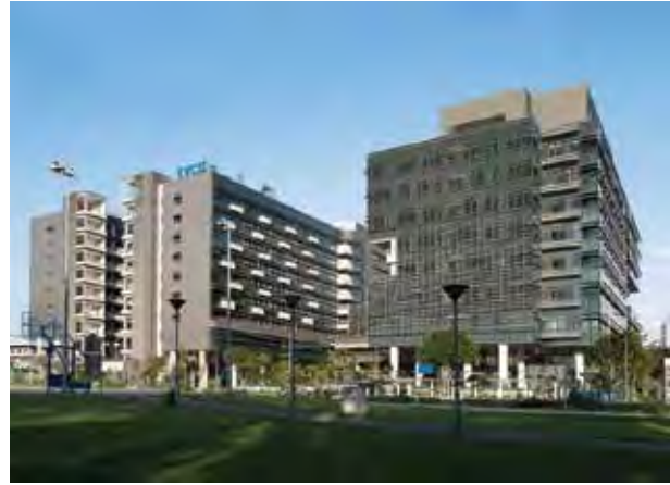
Adopted the use of PCSS and BIM at Yishun Community Hospital (YCH)
