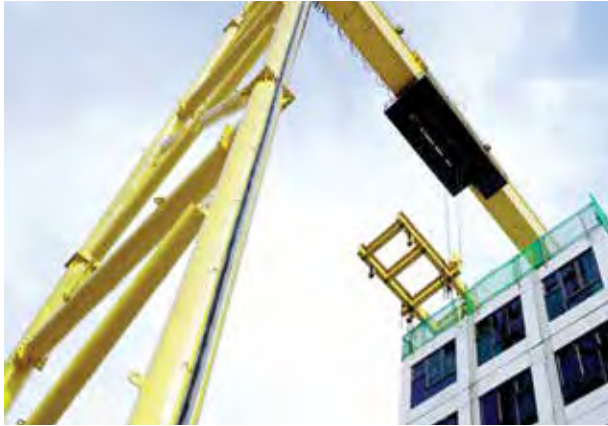
Used concrete PPVC in The Brownstone EC project.
