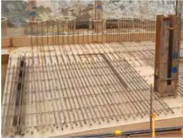
Above: Pioneered the use of carpet reinforcement.
