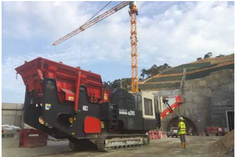
Top, above and left: Contract 6 is seen as a project requiring a multifaceted approach to construction, requiring the use of many different techniques in order to deliver the project on time and within the budget. Here, Sandvik surface drilling rigs, tunnelling jumbos and mobile crushers are being used to help complete the works.
