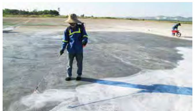
Mapei curing compound being applied to protect the concrete slab surface on the Chu Lai International Airport upgrading project in Vietnam.
