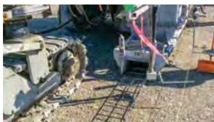
Koyanagawa was tasked to slipform concrete bases for the solar panels to be mounted on. The work had to be completed within 22 days.
