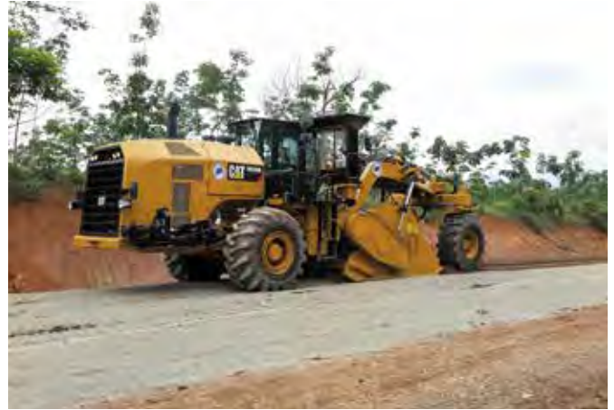
Two Cat RM500B rotary mixers are used for stabilisation of a major coal hauling road in Indonesia.
