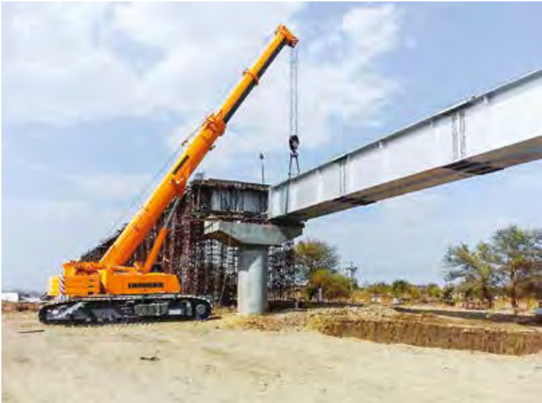
Liebherr LTR 1220 lifts girders on the Nagpur Metro project.
