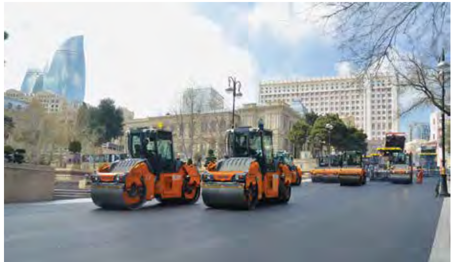
Above: During the construction of the F1 track in Baku, Azerbaijan, Hamm oscillation rollers compacted the asphalt surface efficiently yet with minimal vibration.
