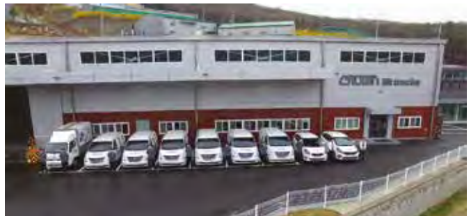
Crown Equipment's new facility in South Korea is located in Icheon, Gyeonggi-do.
