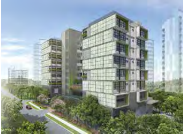
Adopted the use of PPVC at Woodlands Crescent Nursing Home (WCNH).
