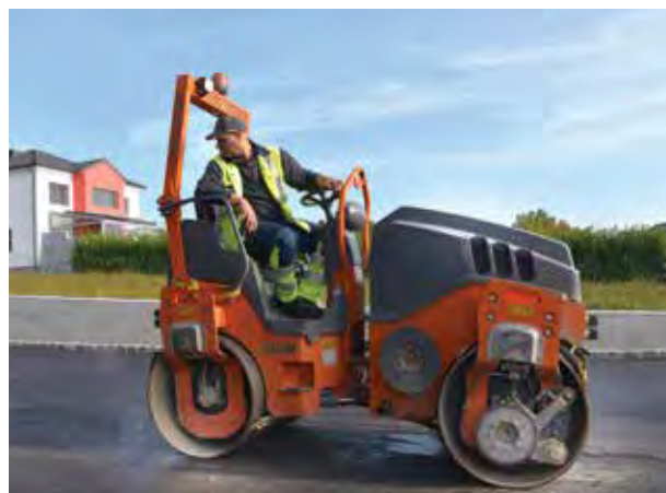
Above: During the construction of the F1 track in Baku, Azerbaijan, Hamm oscillation rollers compacted the asphalt surface efficiently yet with minimal vibration.
