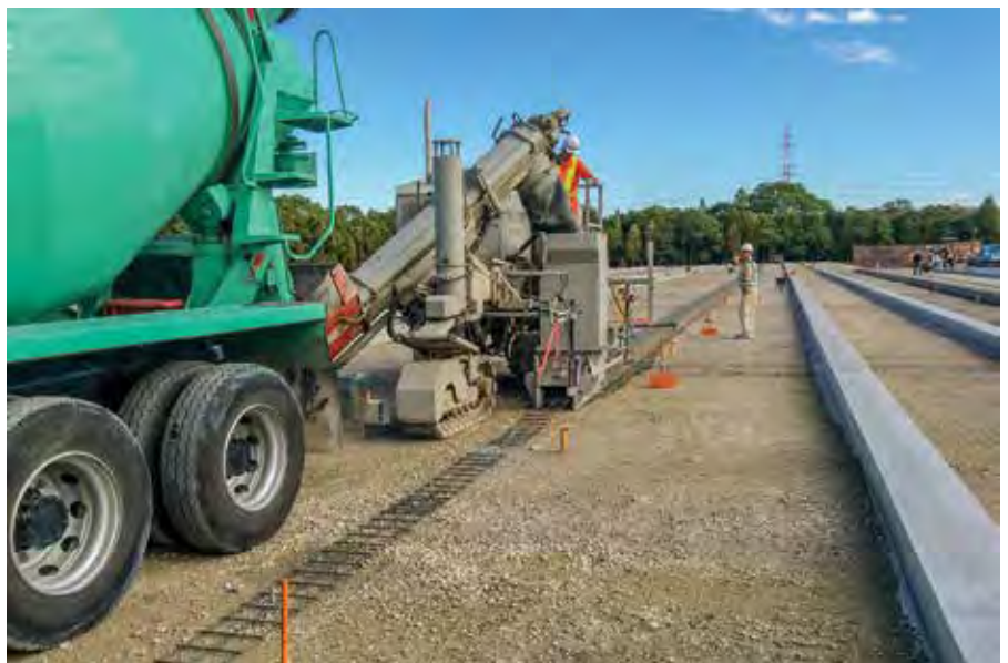
Koyanagawa was tasked to slipform concrete bases for the solar panels to be mounted on. The work had to be completed within 22 days.
