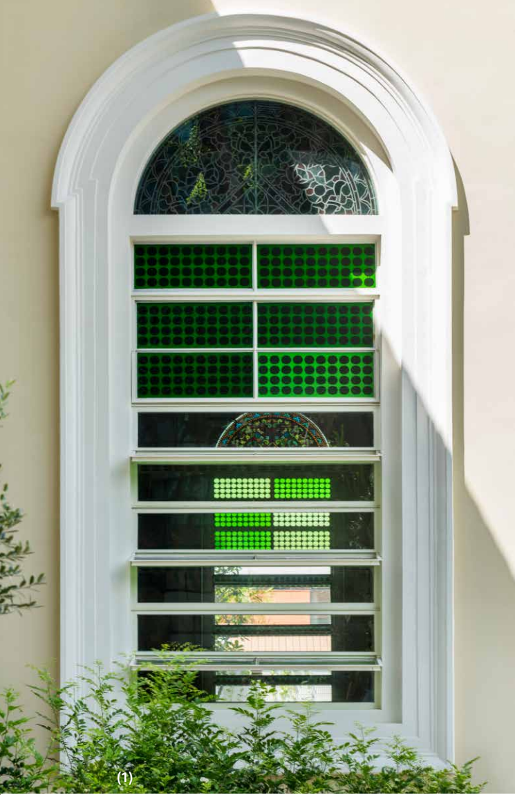
(1) Original mild steel pivoted window with green glass. Photo: © Cathedral of the Good Shepherd (2) 19 th century bell in the steeple restored. Photo: © Cathedral of the Good Shepherd (3) Original encaustic floor tiles in the Rectory. Photo: © Cathedral of the Good Shepherd (4) Stained glass panel at the North transept. Photo: © Vernon Leow of Vital Images, courtesy of Cathedral of the Good Shepherd (5) Pipe organ. Photo: © Studio Lapis
