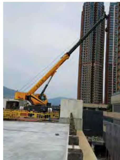
ABOVE AND LEFT: Grove RT550E rough-terrain crane is involved in the upgrading of the Yuen Long MTR station in Hong Kong. The crane works on the station roof to help Yee Hop Engineering hoist up construction materials including steel bars and cement, with loads weighing up to 14 t.
