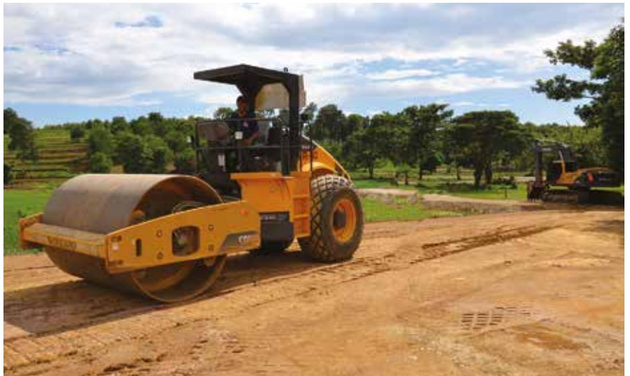
ABOVE: Volvo SD110 single drum compactor being deployed along the AH13 section of the Great Asian Highway project. The section runs 140 km, right through Thailand to the border with Laos.
