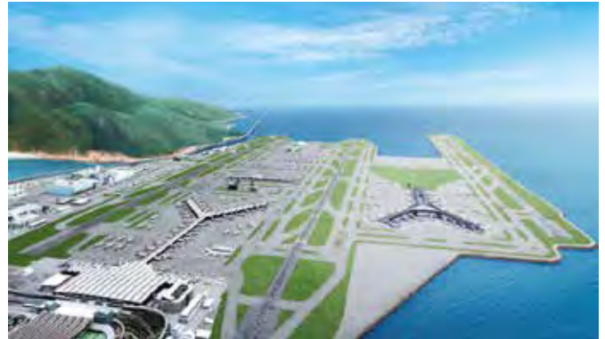
Hong Kong International Airport is expanding its current two-runway system into a three-runway system (3RS).
