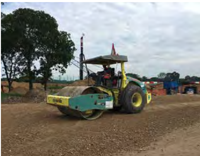
ABOVE AND BELOW: Ammann ASC 110 single drum rollers work on the construction of a new runway at Singapore Changi Airport. The machines are designed with no-rear-axle concept that provides an individual drive for each tyre.
