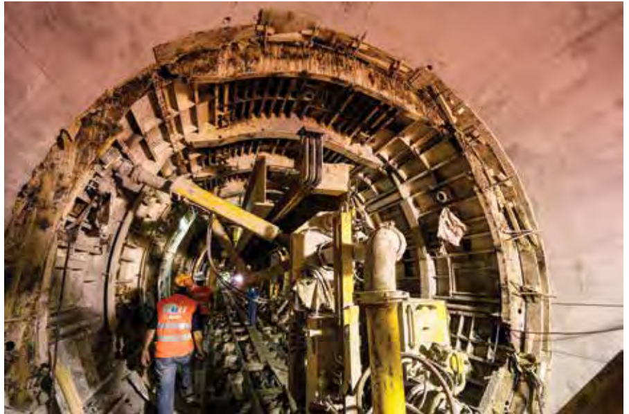
ABOVE: The tunnelling operations were carried out using two full-section EPB tunnel boring machines, designed specifically to operate in areas with water under high pressure.
