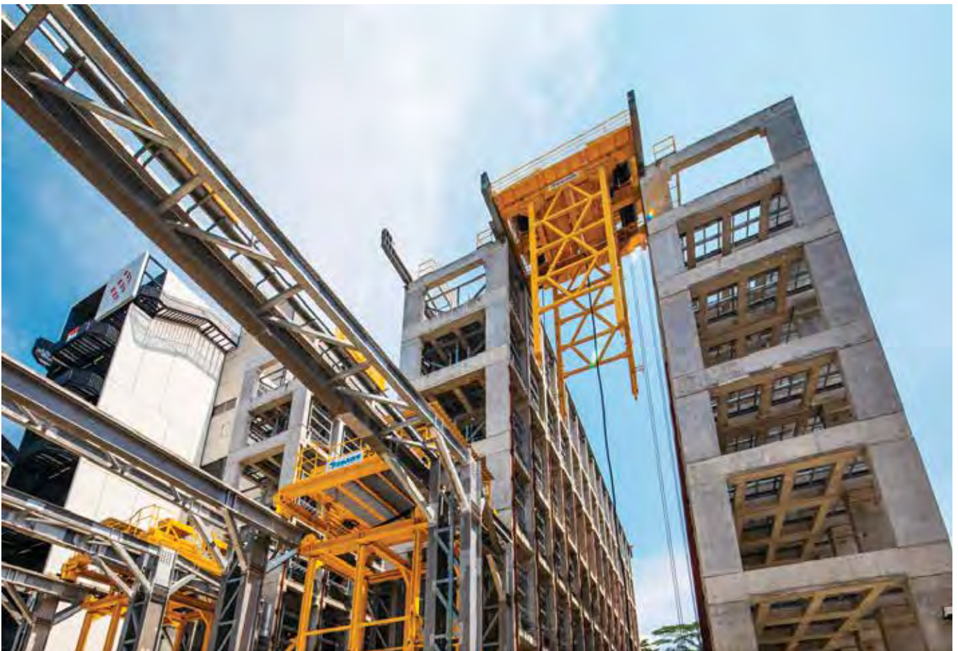
The automated multi-level precast storage facility at Greyform Building has a capacity to accommodate up to 5,800 t of products. This automated system is capable of storing and retrieving an entire rack of precast components onto standard transport trailers. As such, it helps to shorten standby time of transport trailers and improve overall round-trip-time.
