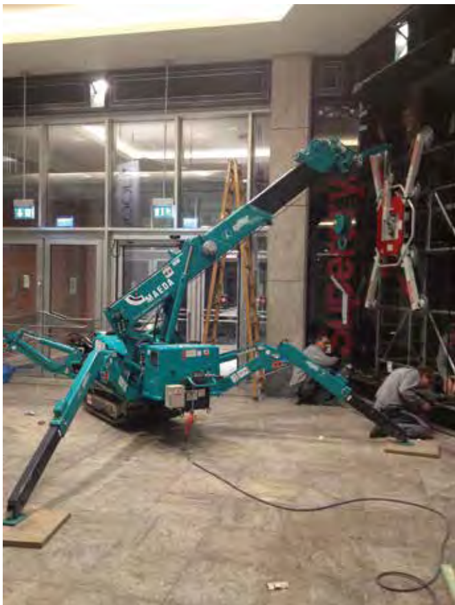
LEFT AND RIGHT: Featuring a modular design, the UPG 600-2 can be adapted to meet job requirements on the construction site. It operates in temperatures ranging from 0° to 40°C, and has the ability to work continuously for up to eight hours.
