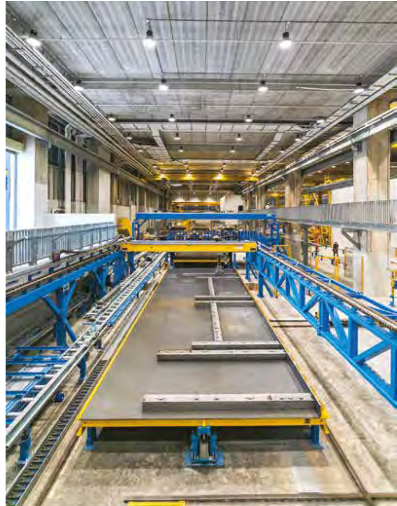
Greyform Building uses automated robotic shuttering for placement of steel magnetic formwork onto the pallet, to create the moulds for precast concrete production.
