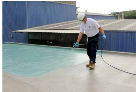
Davco K10 Green Sheet R is a high performance, multi-layer, fabric reinforced, waterproofing system that can be installed using a special spray equipment or roller. It is specially formulated to be fast drying hence increasing productivity and reducing the risk of the membrane being wash out due to the sudden occurrence of rain on during installation.
