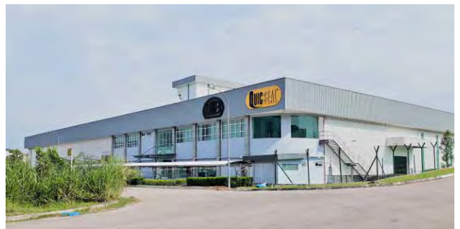
Photo: Courtesy of ARDEX Group and QUICSEAL Construction Chemicals Pte Ltd
