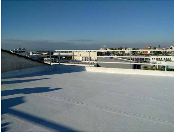
Polyurethane rooftop coating applied on an industrial rooftop.
