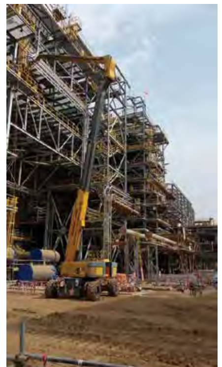
Haulotte aerial platforms have also been involved in Saudi Aramco's new Jazan Refinery and Terminal in Saudi Arabia.
