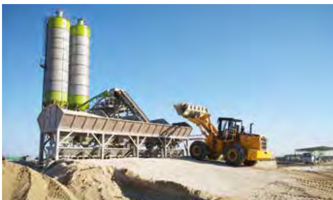
LiuGong machines also participate in the construction of Pakistan PKM expressway, one of the projects under the Belt and Road Initiative.
