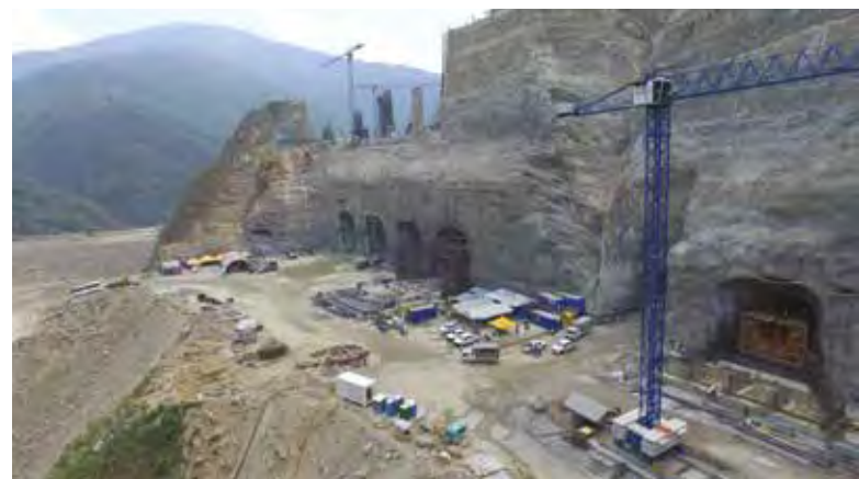
One of the cranes, an 11LC160, is being used to build the intake tunnels, just by the spillway.
