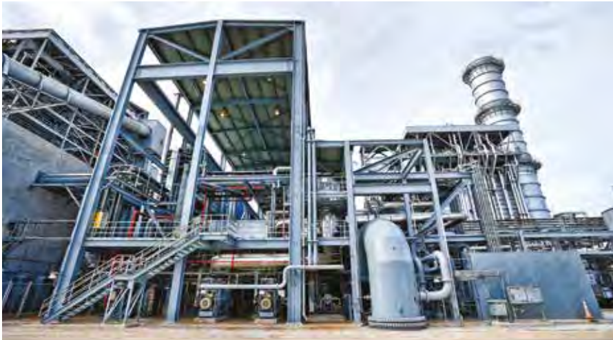
Constructability planning alerted the Glow Phase 5 project team to schedule conflicts prior to construction work starting.
