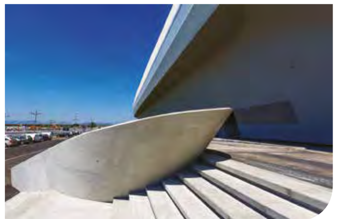
ABOVE RIGHT AND RIGHT: The surfaces were skimmed with Planitop Fine Finish, which was specifically developed for this site. They were then finished off with Malech primer and Colorite Beton paint in a tailor-made RAL colour.
