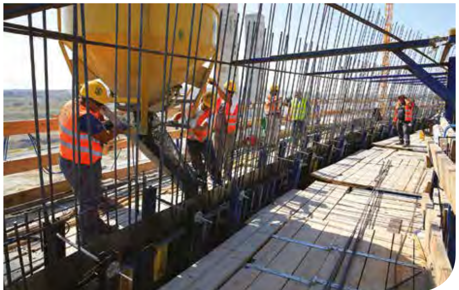
TOP: Construction company Terna uses Doka SK175 cooling-tower formwork on the project. This automatic climbing system is suitable for precision forming combined with short cycle times.
