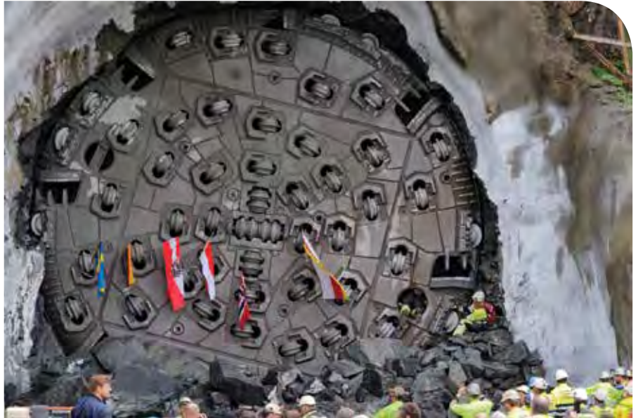
The Ulrikke tunnel boring machine breaks through the target wall. The cutterhead weighs 236 t and was equipped with a total of 62 19-in disc cutters to allow the machine drive through extremely hard gneiss with overburdens of up to 600 m.
