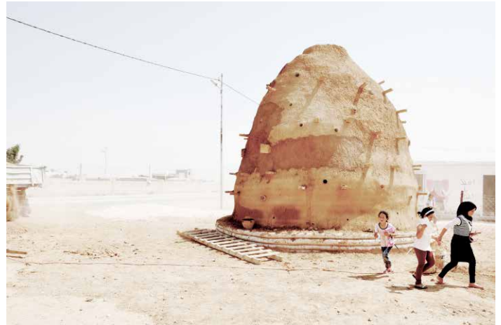
Photo: © Emergency Architecture & Human Rights
