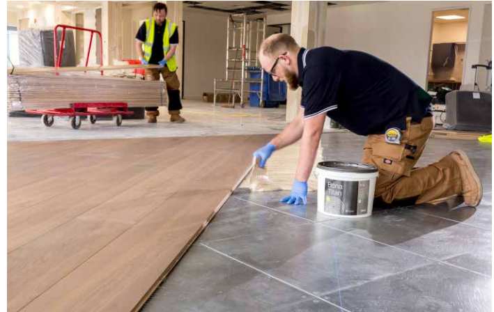
Bona Titan specified to bond wide oak boards to metal subfloor. Photo: © Bona AB
