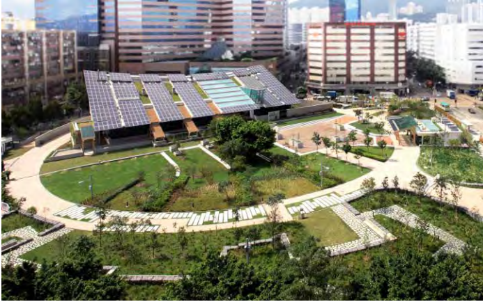
Construction Industry Council – ZCB, Hong Kong – Winner of the 2016 Leadership in Sustainable Design and Performance (Institutional) award. Photo credit: Construction Industry Council
