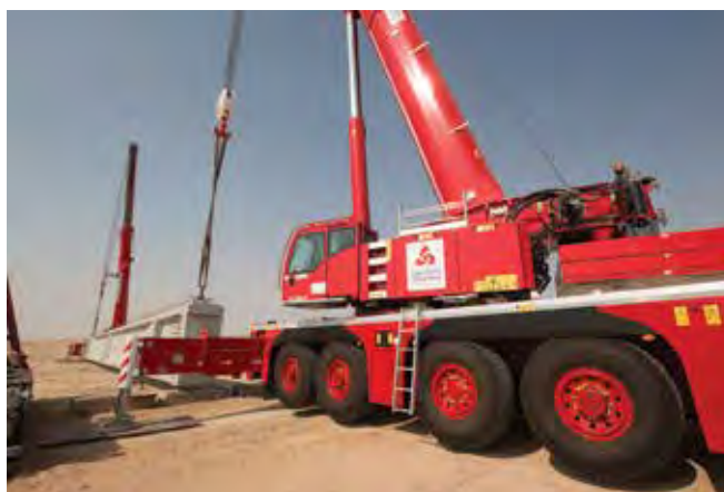
TOP, ABOVE AND LEFT: ILC relied on its new Demag AC 300-6 cranes on the Sheikh Jaber Al Ahmad Al Sabah Causeway Project in Kuwait. The cranes had to lift precast concrete components and place them at their pre-planned position. As the elements weighed 105 t each, were approximately 37 m long, 1 m wide and 2.3 m tall, the work was best done with a tandem lift.
