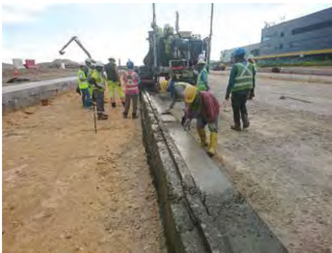
LEFT: Initial practice trial was also conducted for paving team and supervisors, so that they could understand the workability of low slump concrete's challenges.
