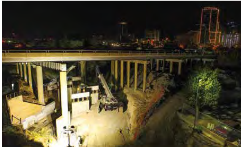
ABOVE AND LEFT: The TCC-2500 works on the project together with the Link-Belt TCC-1100 crawler crane.
