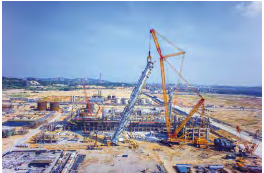
ABOVE, LEFT, BOTTOM AND BOTTOM LEFT: The 4,000-t XCMG XGC88000 crawler crane carries out a major lifting operation at one of petrochemical industrial parks in Dalian, China. The crane has a maximum load moment rating of 88,000 tonne-metres, and through a combination of components, it can be transformed into a 2,000-t unit.
