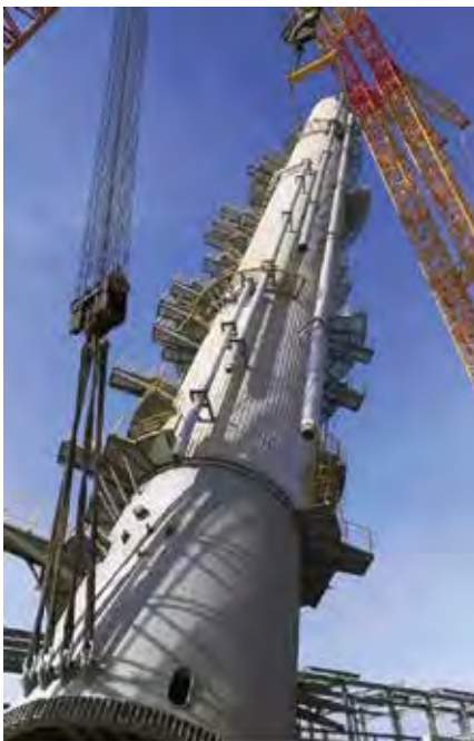
ABOVE, LEFT, BOTTOM AND BOTTOM LEFT: The 4,000-t XCMG XGC88000 crawler crane carries out a major lifting operation at one of petrochemical industrial parks in Dalian, China. The crane has a maximum load moment rating of 88,000 tonne-metres, and through a combination of components, it can be transformed into a 2,000-t unit.
