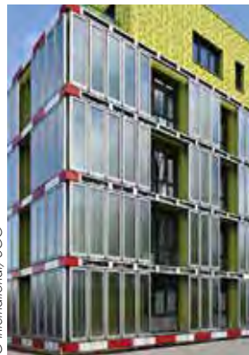
BIQ HAMBURG: Facade panels filled with algae contribute to net-zero energy buildings.
