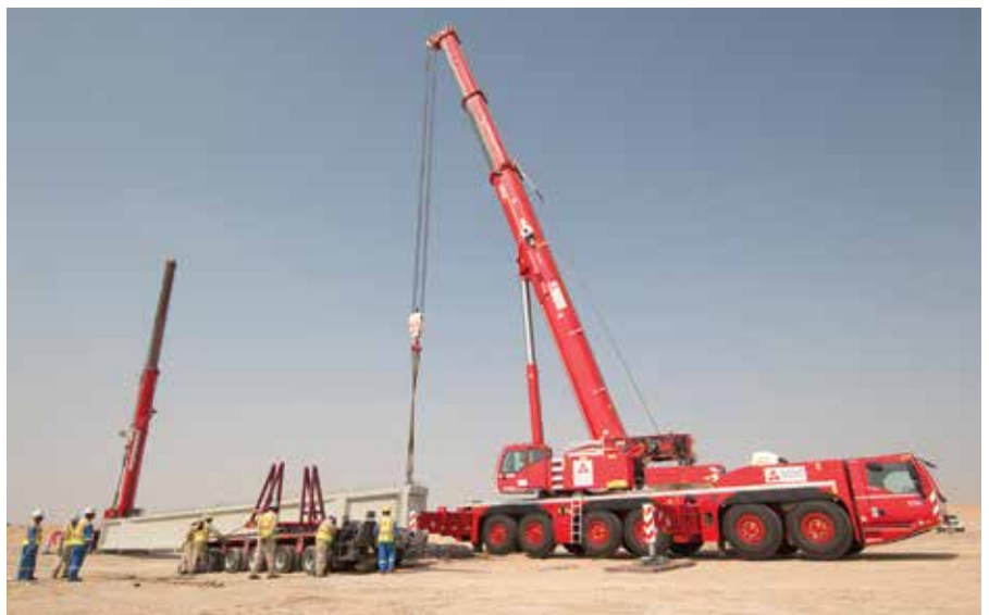
TOP, ABOVE AND LEFT: ILC relied on its new Demag AC 300-6 cranes on the Sheikh Jaber Al Ahmad Al Sabah Causeway Project in Kuwait. The cranes had to lift precast concrete components and place them at their pre-planned position. As the elements weighed 105 t each, were approximately 37 m long, 1 m wide and 2.3 m tall, the work was best done with a tandem lift.
