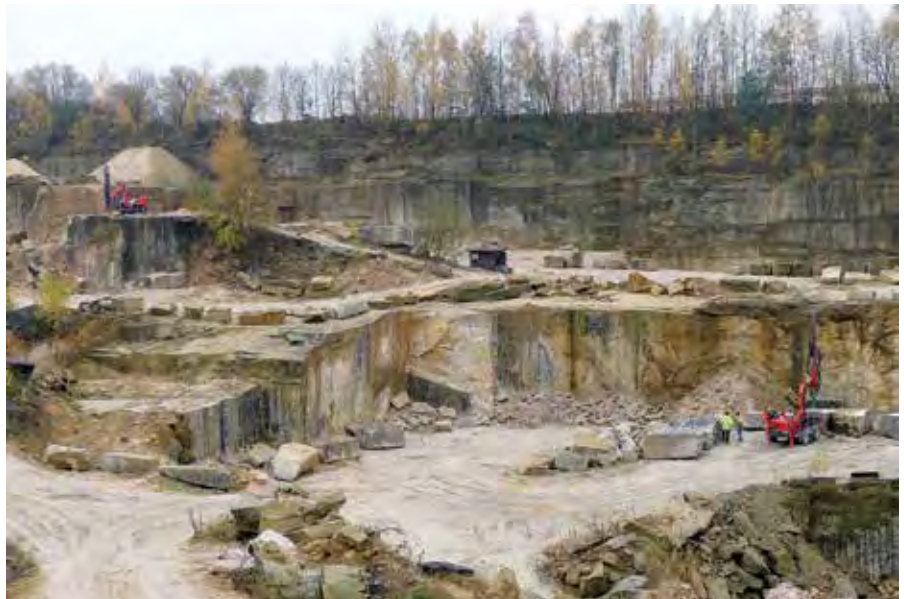
Sächsische Sandsteinwerke employs a total of five Sandvik drill rigs. Two of them, a Commando DC302 and a Commando DC130Ri, are currently used for block extraction on different beds at the Lohmen quarry.
