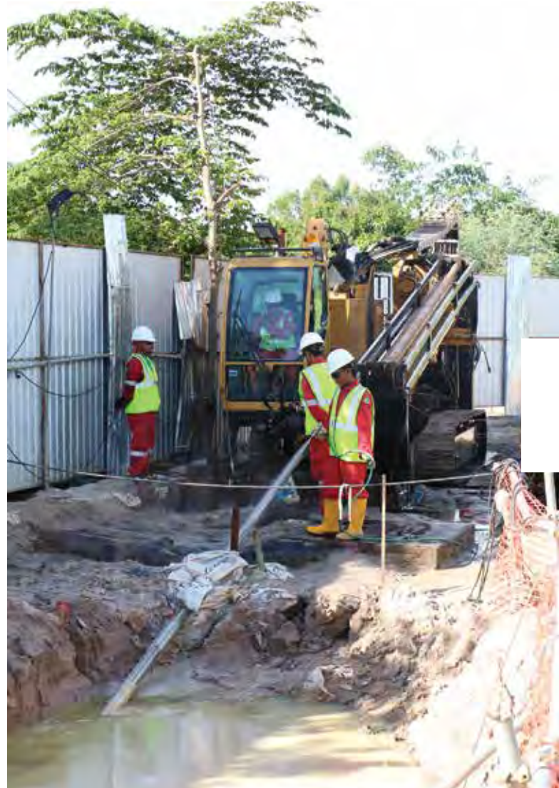
ABOVE AND BELOW: The Vermeer D130x150S drill rig offers 59,000 kg of pullback force and 20,337 Nm of torque.
