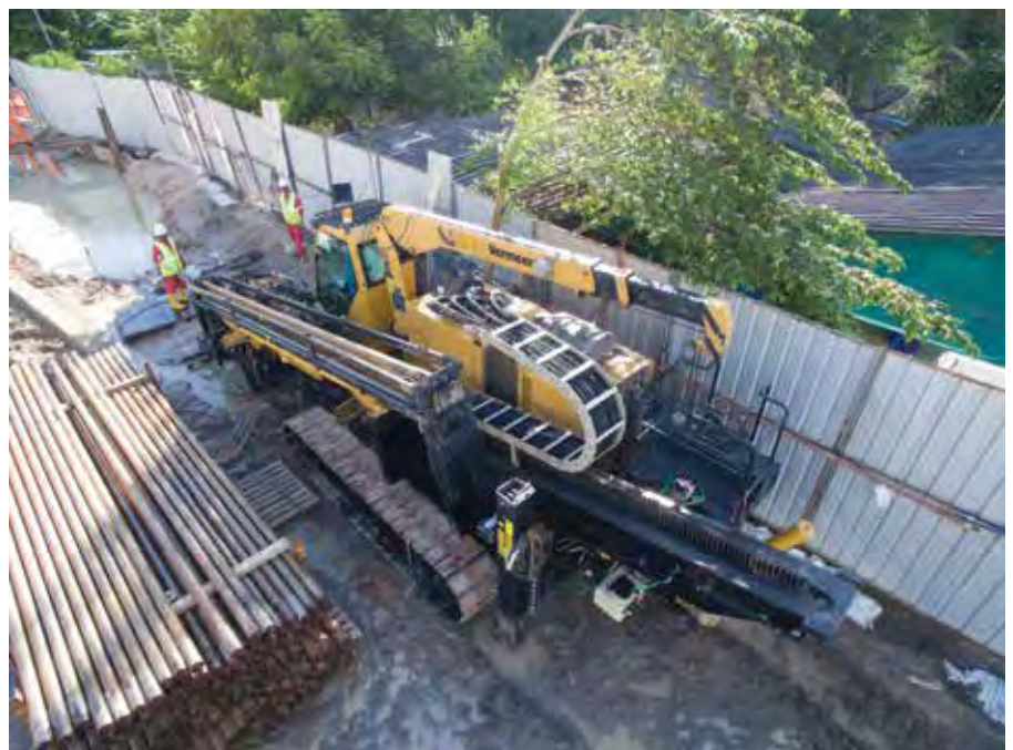
BELOW LEFT: The D220x300S is able to stage five rods at one time, increasing boring efficiency by minimising rod loading time.
