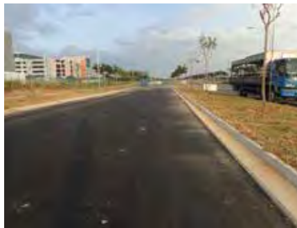
BELOW AND BOTTOM: After a number of trials, the project began and was completed in January 2018. These images show the completed curb and base set for the asphalt course to be laid. The turf has also been completed.
