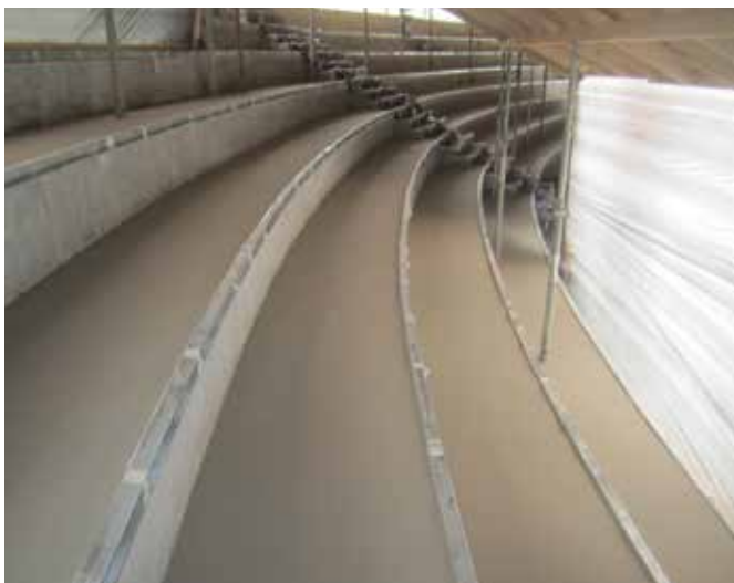
ABOVE AND LEFT: Mapei products have been used to repair and level the concrete, prepare the substrates of the stands and for installing natural stone.
