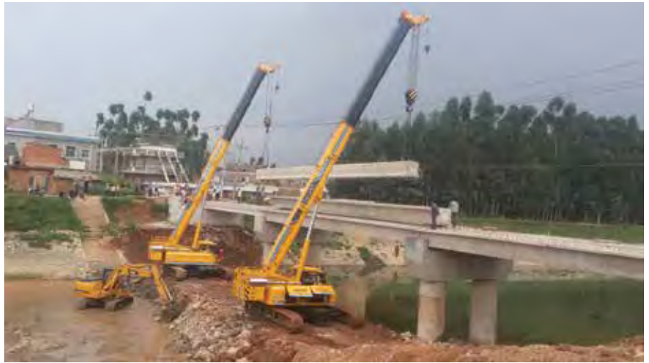
ABOVE AND LEFT: The XCMG XGC55T telescopic crawler crane has a maximum lifting capacity of 55 t, with a five-section boom. It is designed for various applications.
