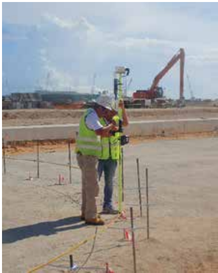
ABOVE: Surveyor marks out points first and then cross checks with Field Rover again, after stakes are setup during training.
