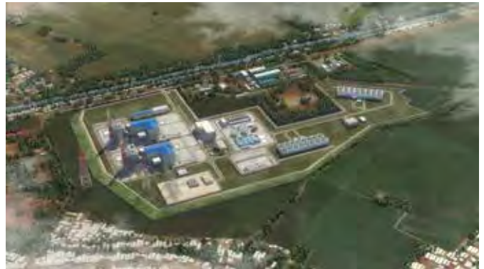
The new 1,760 MW Jawa 1 power plant in Cilamaya, Indonesia, is expected to be the biggest combined cycle power plant in Southeast Asia.
