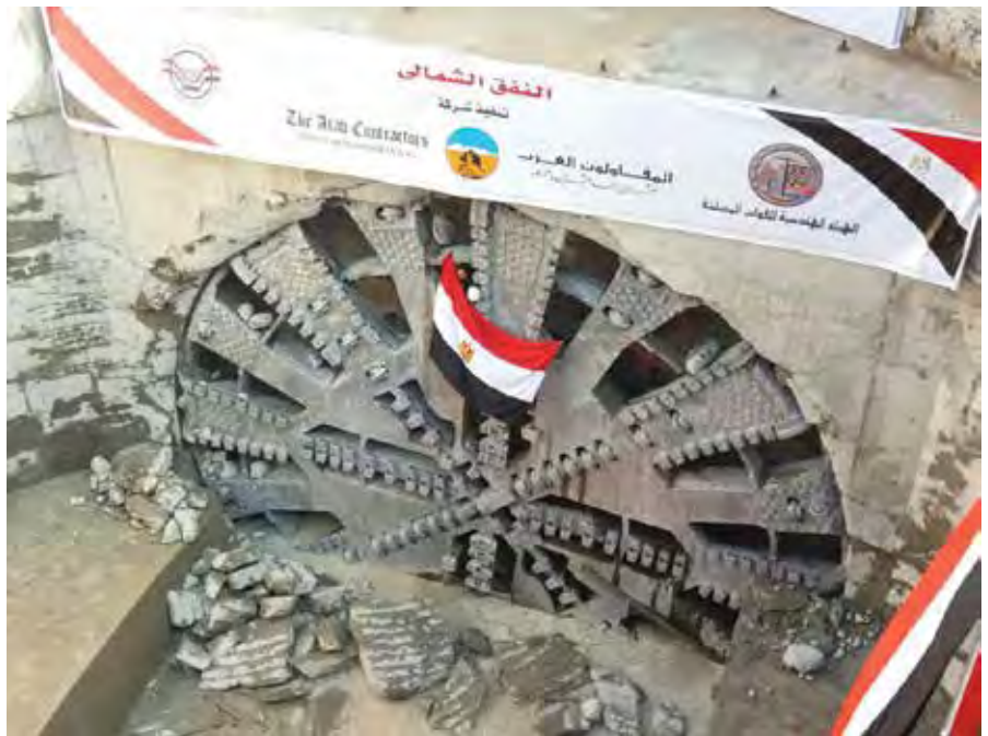
ABOVE: In mid December 2017, the Herrenknecht Mixshield S-959 celebrated its final breakthrough. The TBM drove one of the tunnel tubes at Port Said with top performances of up to 128 m per week.
