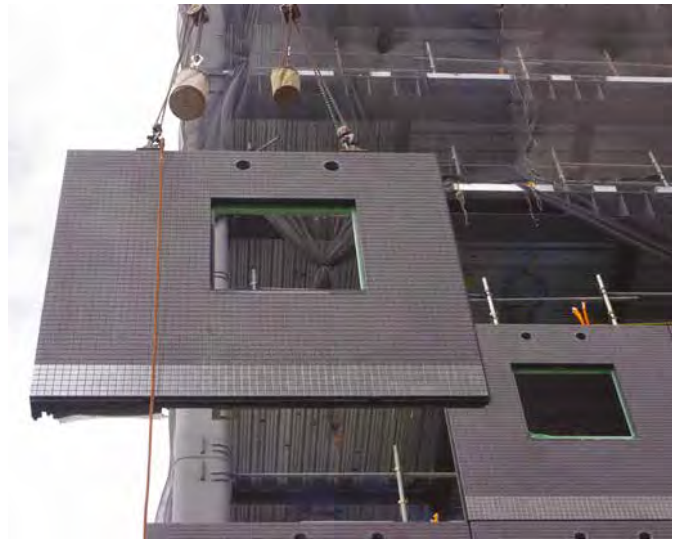
Kanacrete lightweight architectural precast non-structural wall panels provide faster build speeds as well as greater design opportunities with compatibility for various finishes to meet specific construction project needs.
