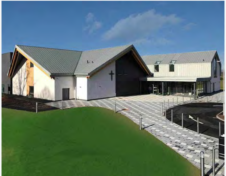
Kentec’s Taktis Technology Platform helps protect an iconic new £4.7 million community hub development for Scotland’s Dumfries Baptist Church.
