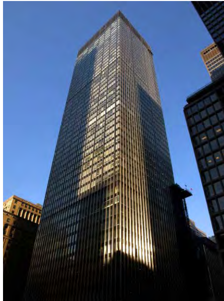
270 Park Avenue in New York City. Photo: © Marshall Geromette
