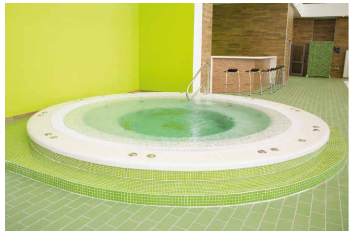
The surfaces of the hot tub in the sports complex were waterproofed with MAPELASTIC.
