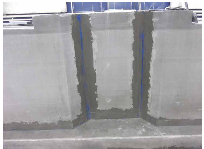
MAPEBAND alkali-resistant rubber tape was used in the pool for the elastic waterproofing of joints between walls and between walls and floors.
