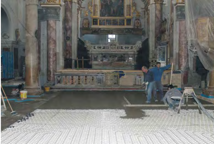
TOPCEM PRONTO was used to build heated screeds.
