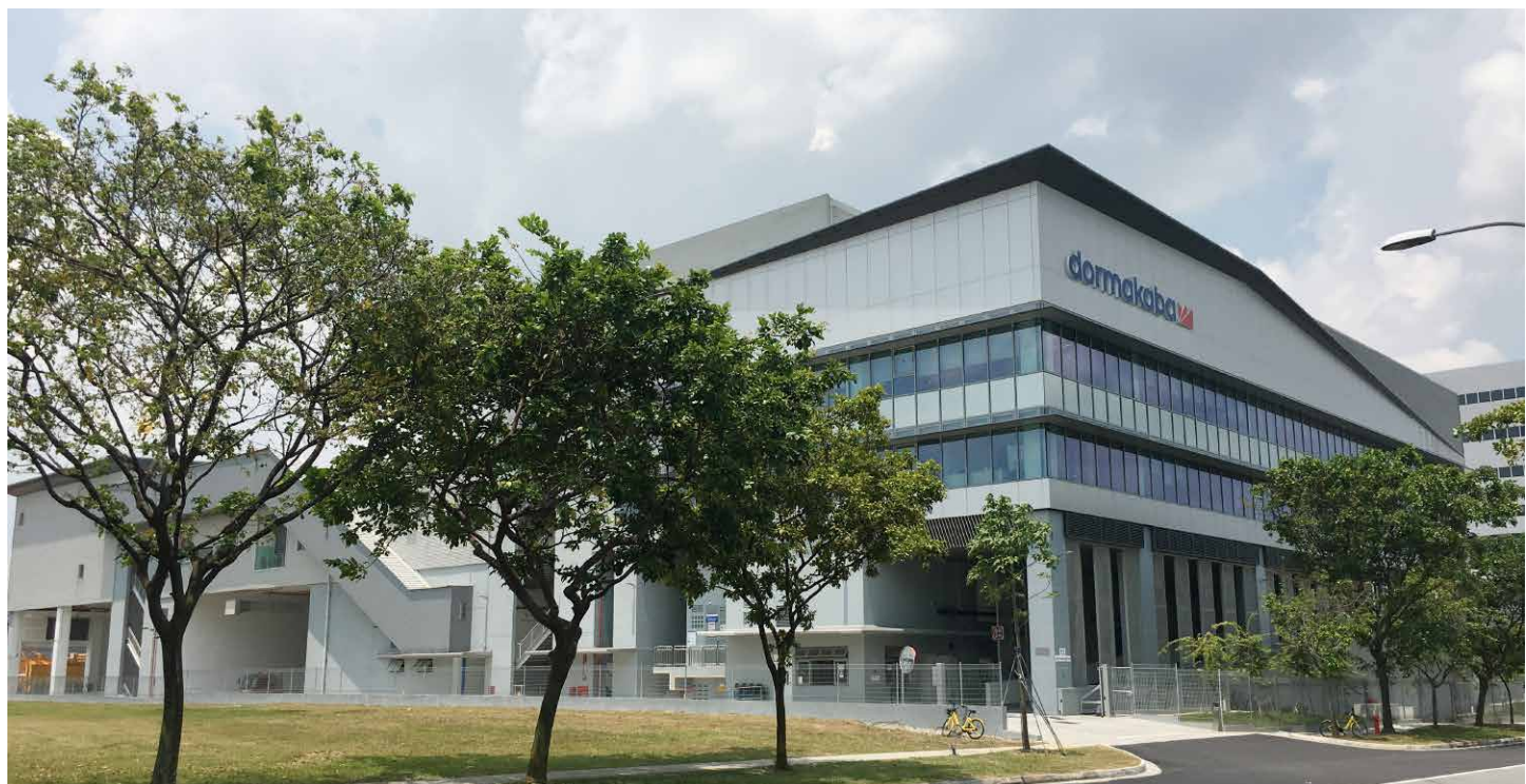
dormakaba's new facility in Singapore.
