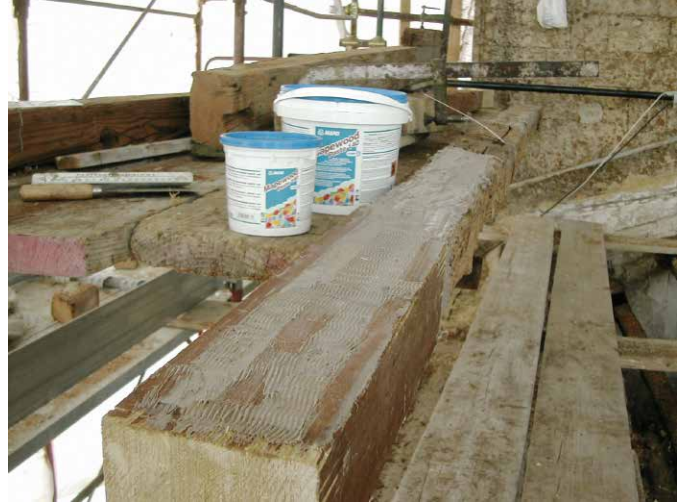
Repairing the beams with MAPEWOOD PASTE 140 .
