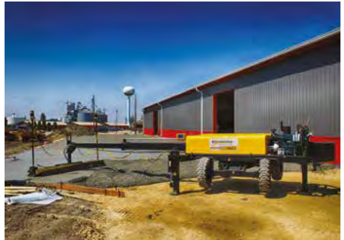
Ligchine will showcase its wireless remote controlled, boom operated, concrete screeding machines, which offer 3D paving capabilities.
