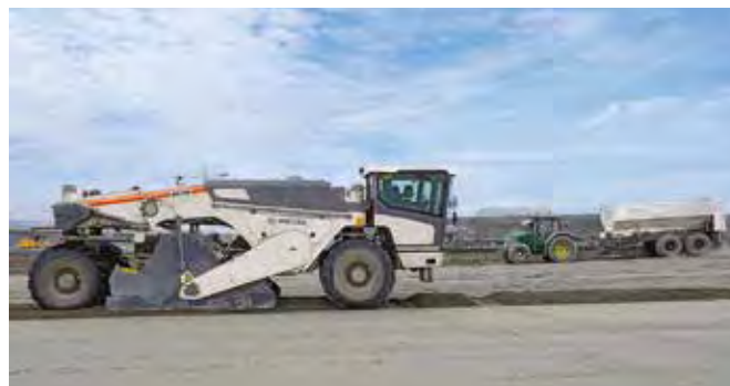
Wirtgen soil stabilisers were involved in the earthworks.
