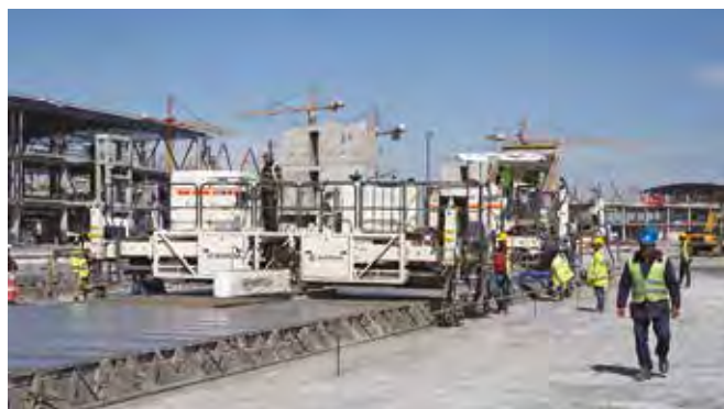
Wirtgen slipform pavers are used for paving concrete taxiways.
