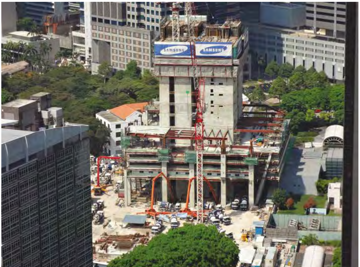
Skidmore, Owings & Merrill, a US-based architecture firm, designed the skyscraper, which was built using the top-down construction method - allowing the basement and aboveground levels to be built simultaneously. Contractor on the project was Samsung C&T.
