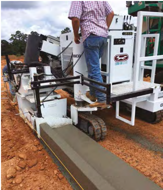
Curb Fox CF 5000-T slipform paver can handle the full range of curb, curb and gutter, channel, sidewalk (up to 3 m wide), and median barrier (up to 1.1 m high).
