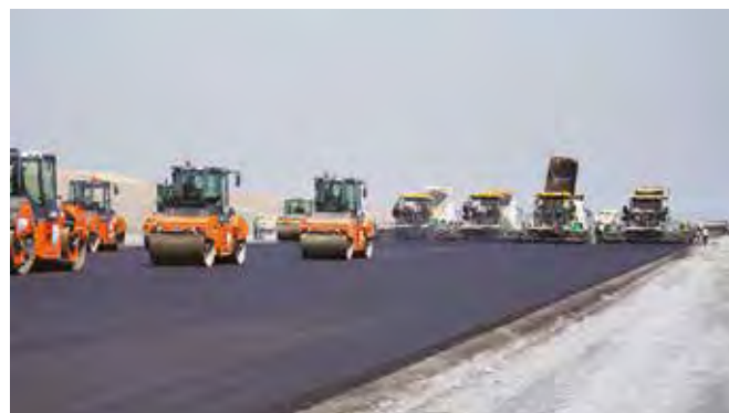
Vögele road pavers and Hamm compactors and tandem rollers are deployed for the asphalt paving job.
