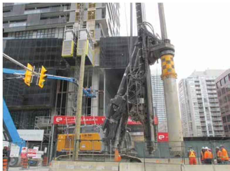
TOP AND MIDDLE: Eglinton Station will be an underground station located at the busy Yonge Street and Eglinton Avenue intersection. The cut-and-cover construction method is being used here, which means excavation is performed then covered with wooden decking while crews continue digging and building underneath.
