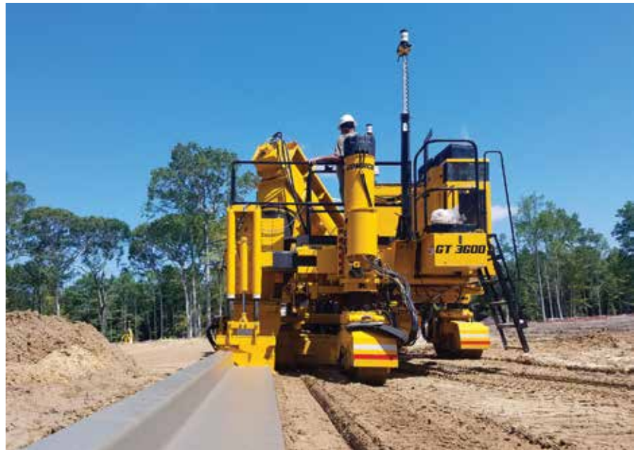
A Gomaco Xtreme GT-3600 slipforms curb and gutter on a cul-de-sac in a residential development. The Xtreme system adds G+radius software with slew drives, smart-sensored hydraulics and intelligence to the GT-3600 paver.
