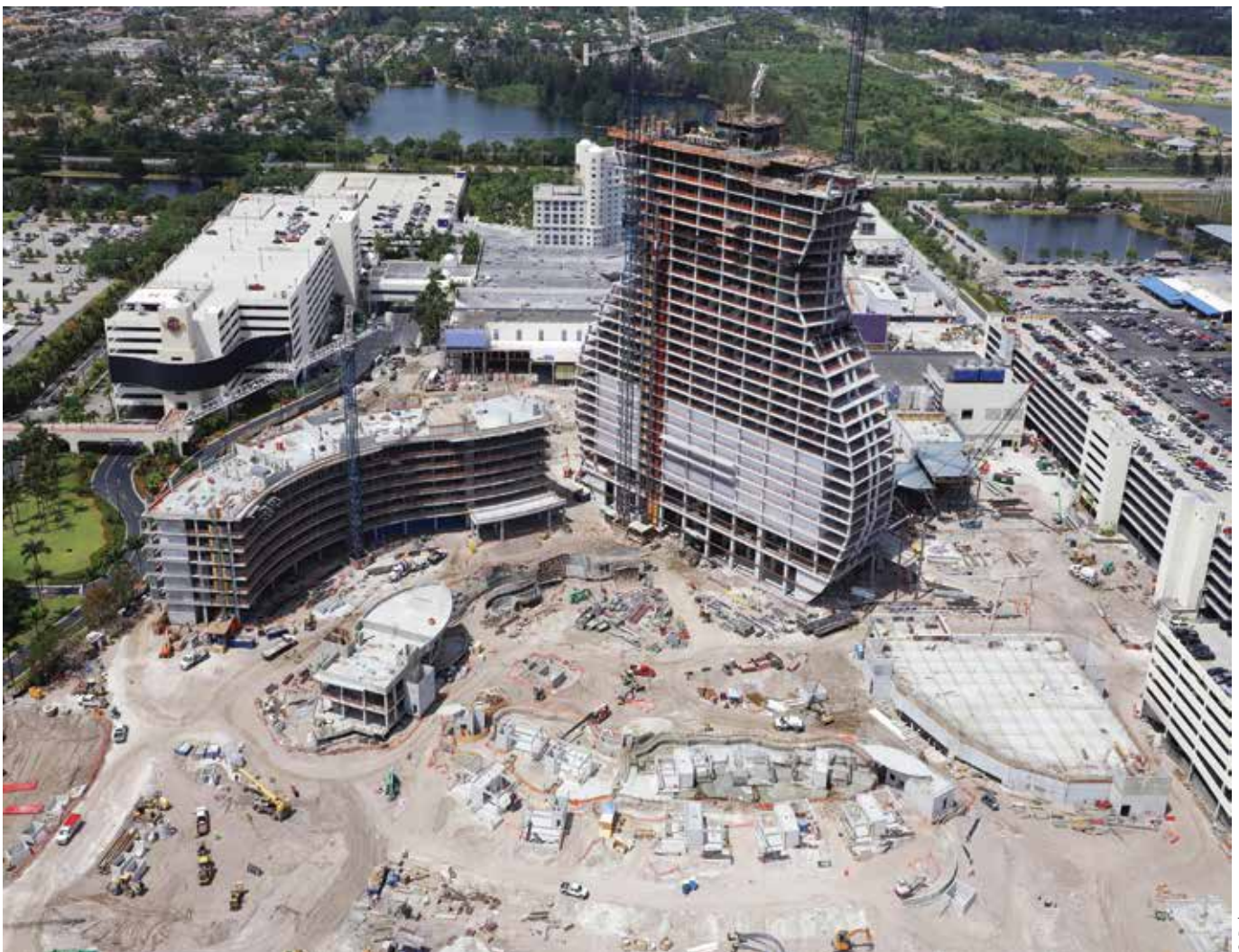
Doka has supplied a variety of formwork systems to help complete the project.
