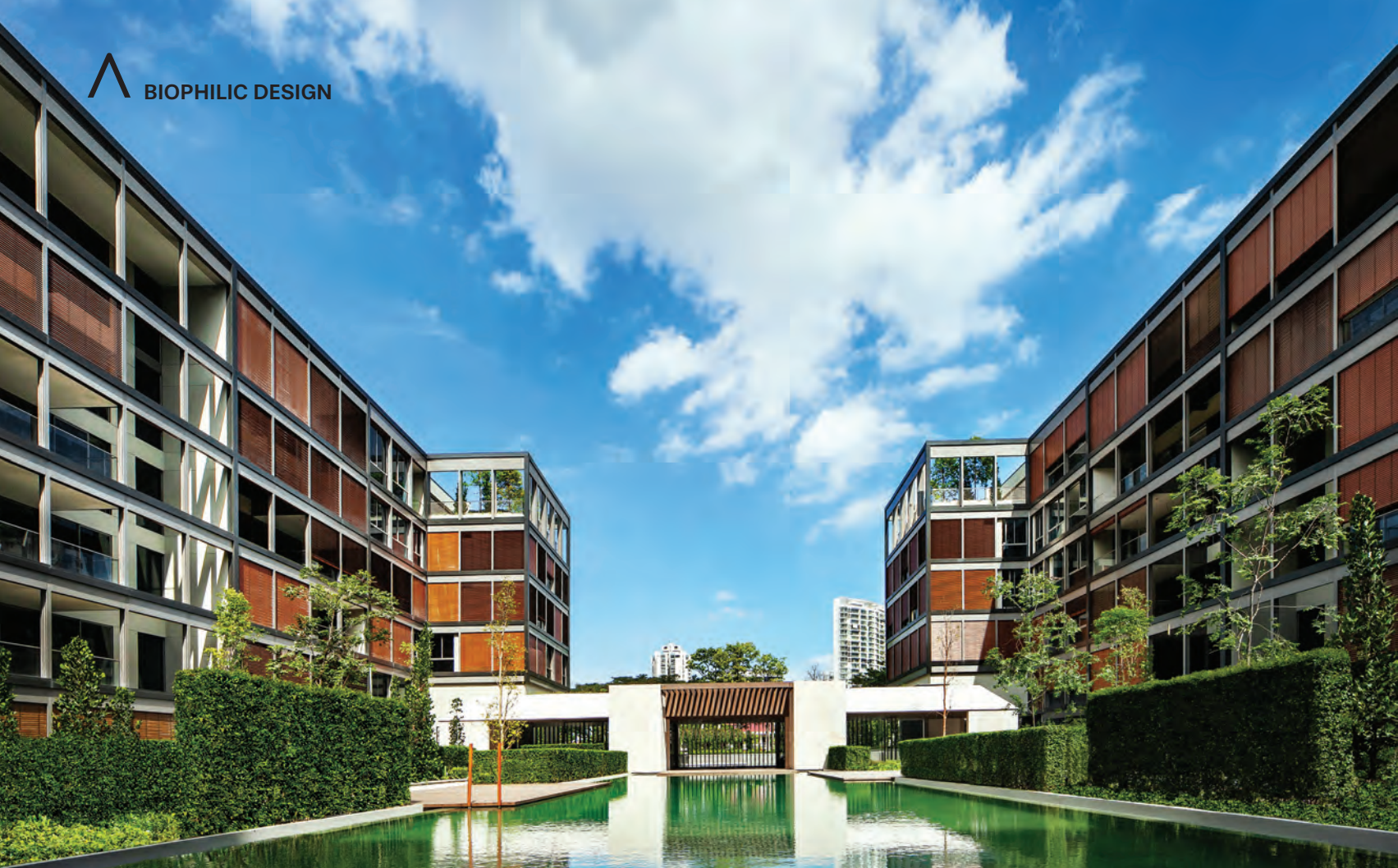
Axial view of MeyerHouse to forested park. Photo credit: Patrick Bingham-Hall
