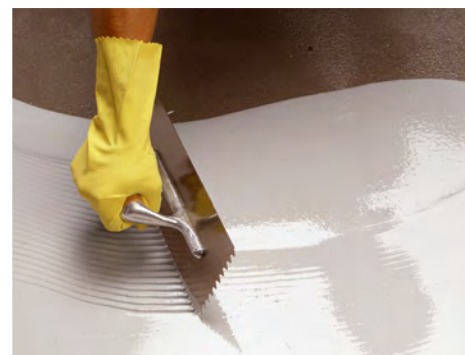
Application with Mapefloor CPU
